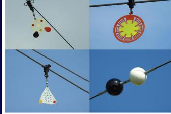
Almost 270 km of power lines were identified as a priority for increasing the visibility via installation of bird flight diverters and use of insulated conductors.
